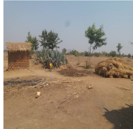
Latrine designs in the Catchment often not roofed thus prone to collapse and they fill up with water as well as the raising water table (Photo by CADECOM Blantyre)
