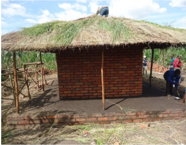
HEAPED ROOF WITH BOUND GRASS TO PROTECT FROM STRONG WINDS
