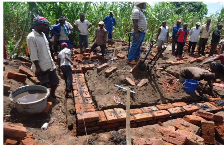
Thick Waals being protected with Clay
